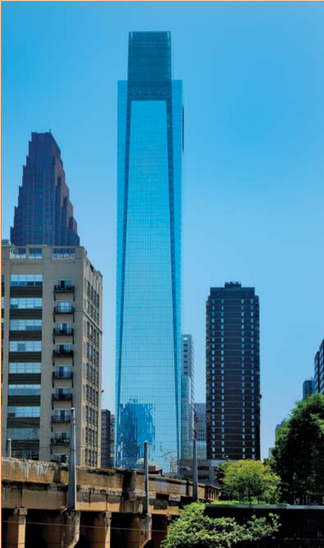
Figure 7.3 Comcast Center's glass façade blending in with the sky. One thousand birds per year have been estimated to die striking this and adjacent buildings.
