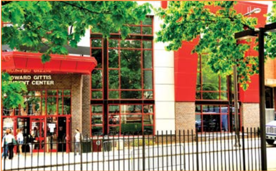
Figure 7.5 Temple University’s Howard Gittis Student Center, with windows that reflect images of street trees, promoting collisions by birds. In 2011, 1,200 birds including thirty-one species were recovered around Temple’s campus buildings, including this building.
