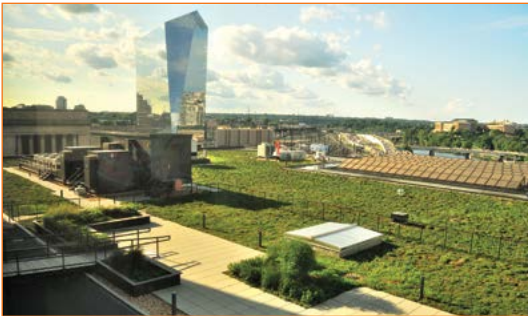
Figure 29.3 Green roof on top of PECO (Philadelphia Electric Company) building in Center City.
