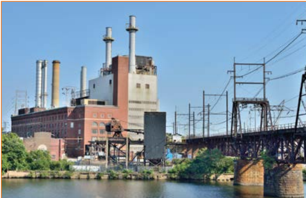
Figure 21.13 Cluster of three power plants on the Schuylkill River at Christian Street, a few blocks south of Center City. View is from the Schuylkill Expressway. A cooling water intake structure along the shoreline draws water from the river. Fish sucked through a pipe strike a screen that diverts them into a trash trench for disposal offsite.
