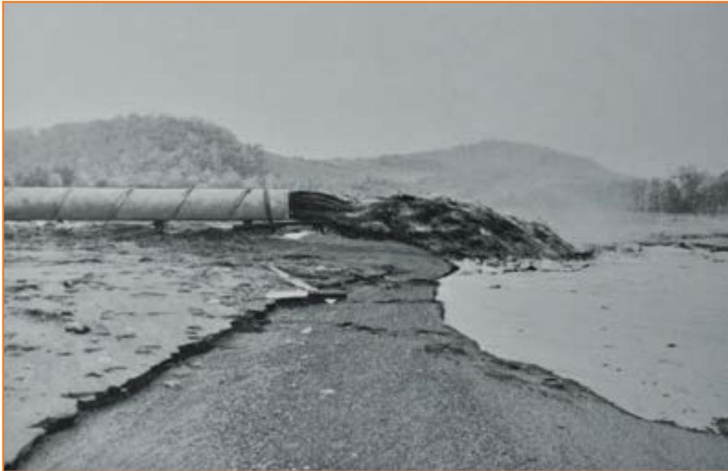
Figure 20.4 Schuylkill River desilting project discharging dredged materials into an impounding basin upstream at Stouds Ferry, Berks County. (From *The Schuylkill River Desilting Project, Final Report of the Schuylkill River Project Engineers*, 1 July 1951<sup>17</sup>)
