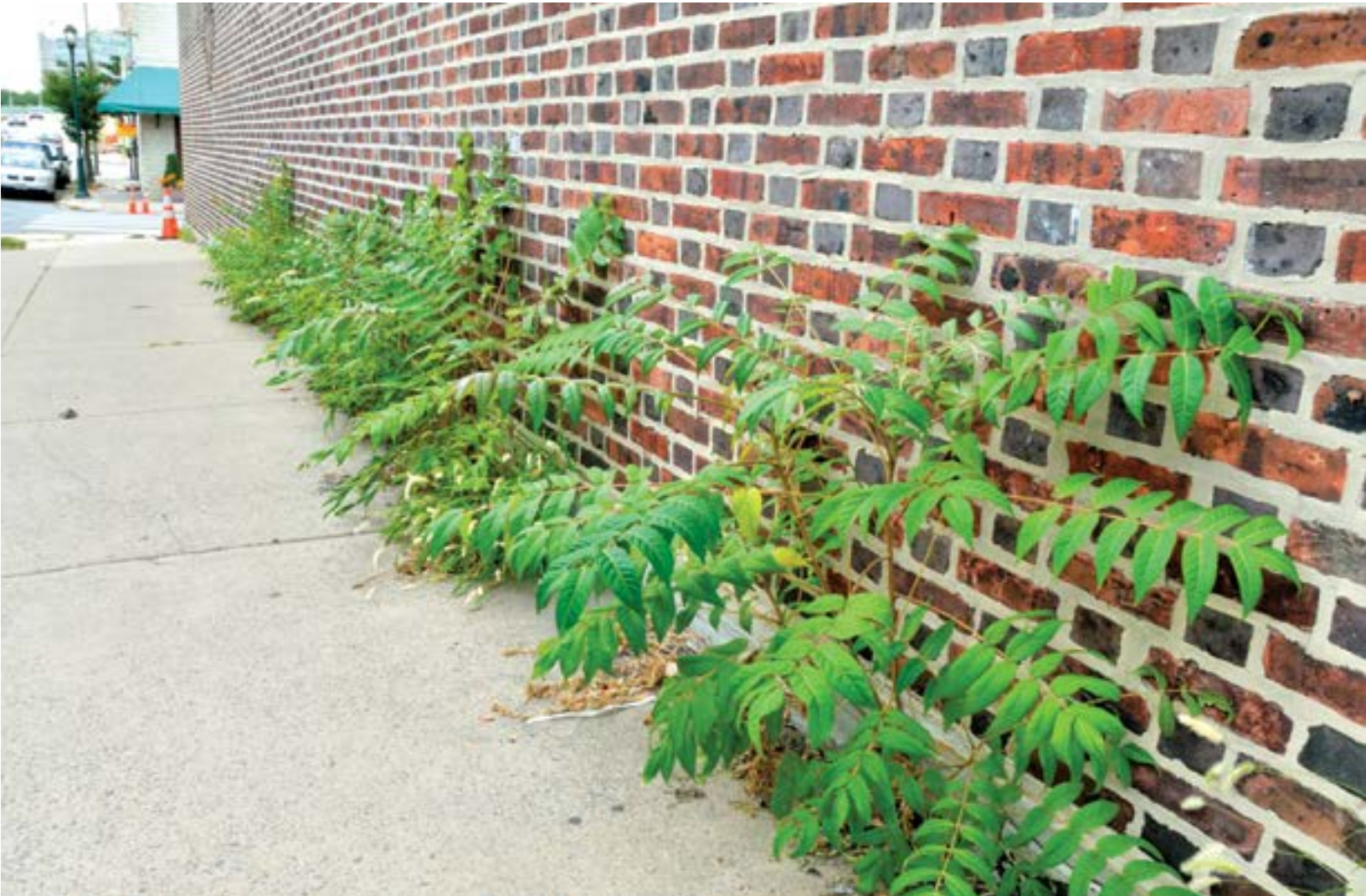
Figure 5.3 Colony of ailanthus saplings outside O'Connor Swimming Pool on Lombard Street. They are sprouting from roots tracking along the crack at the base of the wall.
