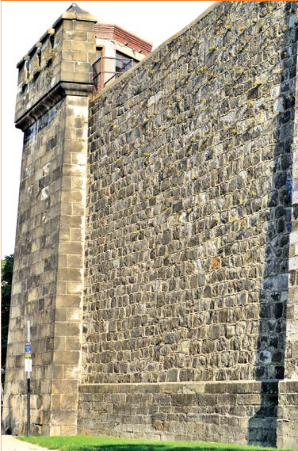
Figure 18.2 Eastern State Penitentiary, north wall, viewed looking east. At this distance, ferns growing in the wall are practically invisible.
