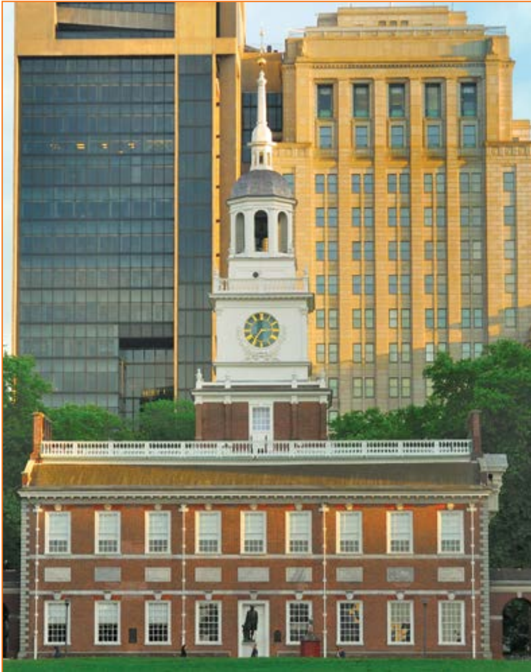
Figure 1.3 Independence Hall, constructed with bricks made from clay deposited a few blocks away by glacial meltwater.
